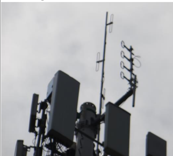
On the right is the installed 2M antenna.
