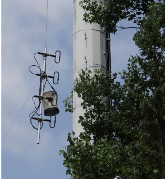
This is the new 2M antenna on its way to the top of the tower.
